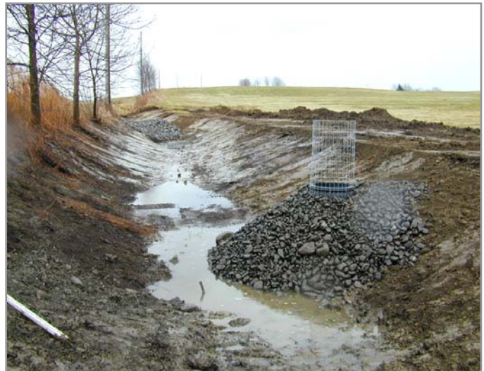
Grate installed on a drainage inlet.
