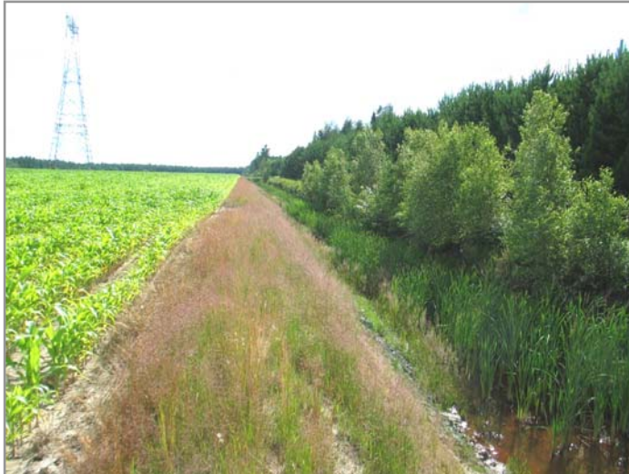
Basin built in an agricultural ditch.
