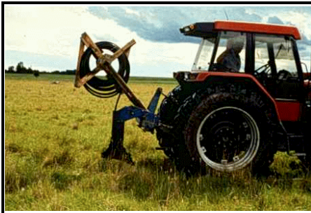
Plowed Installation of Shallow-Buried Pipe From "Pasture Water Systems for Livestock", Alberta Agriculture, Food and Rural Development, http://www.agric.gov.ab.ca/agdex/400/400_716-3.html
