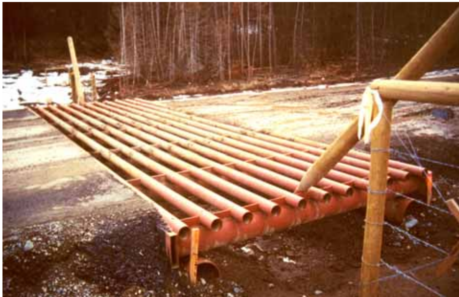
Figure 13 Spring-type Temporary Cattle Guards
