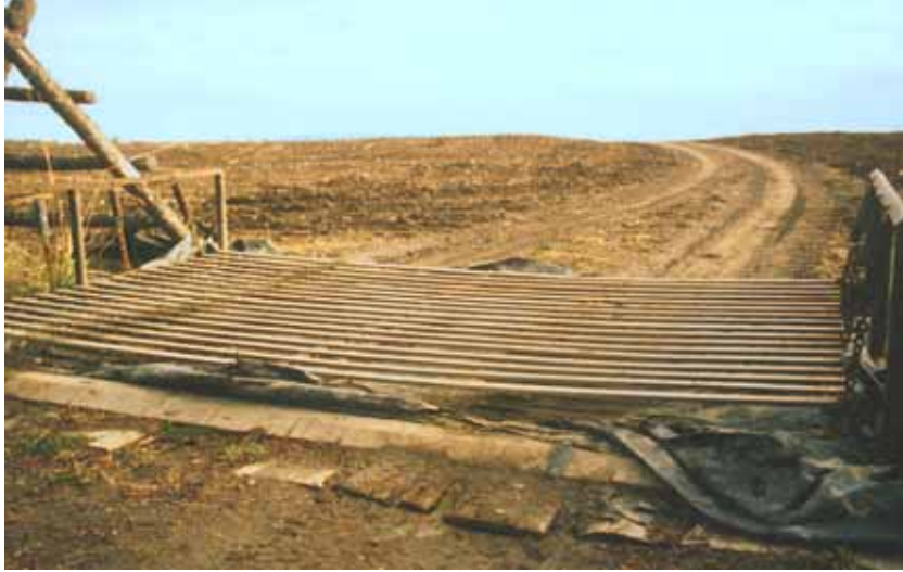
Figure 12 Spring-type Temporary Cattle Guards
