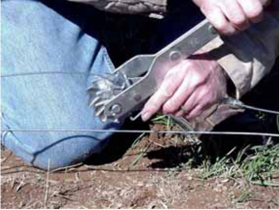
Figure 12 Tightening brace wire
