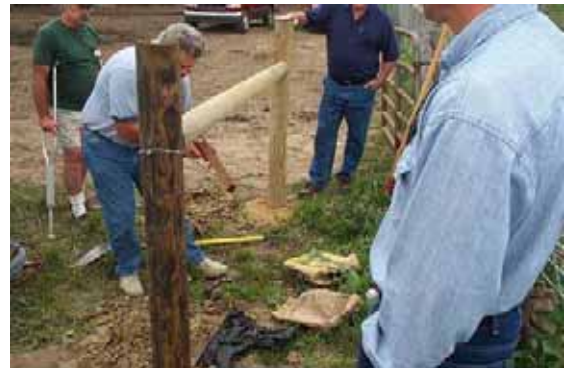
Figure 4 Tightening brace wire
