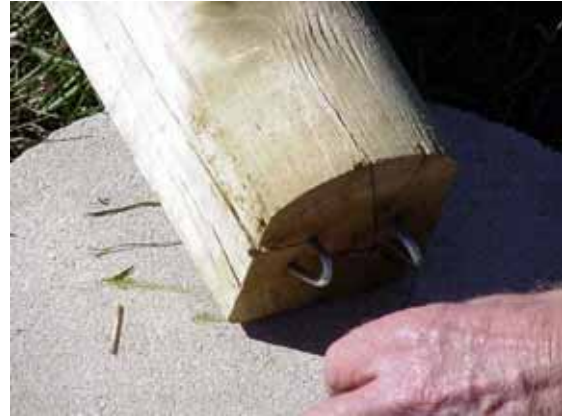
Figure 9 Attaching brace wire
