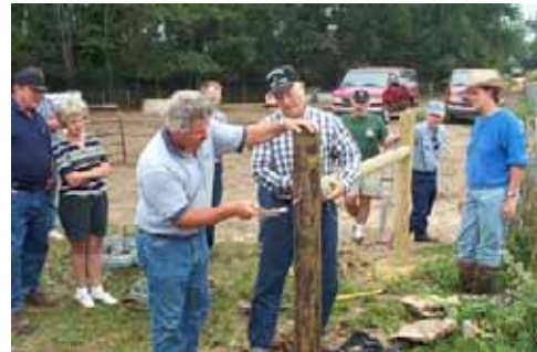
Figure 3 Attaching brace support
