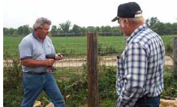
Figure 2 Drilling hole to attach brace support
