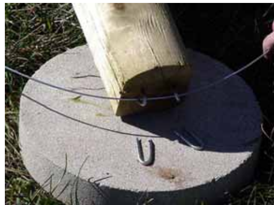
Figure 10 Attaching brace wire
