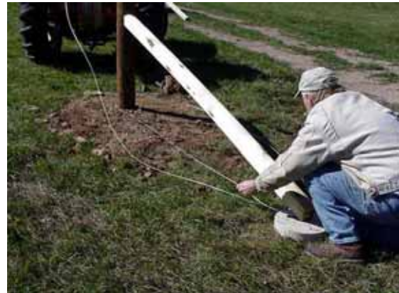
Figure 11 Adjusting brace wire
