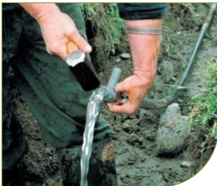
USE 100-PSI PIPES OF THE RIGHT DIAMETER.
