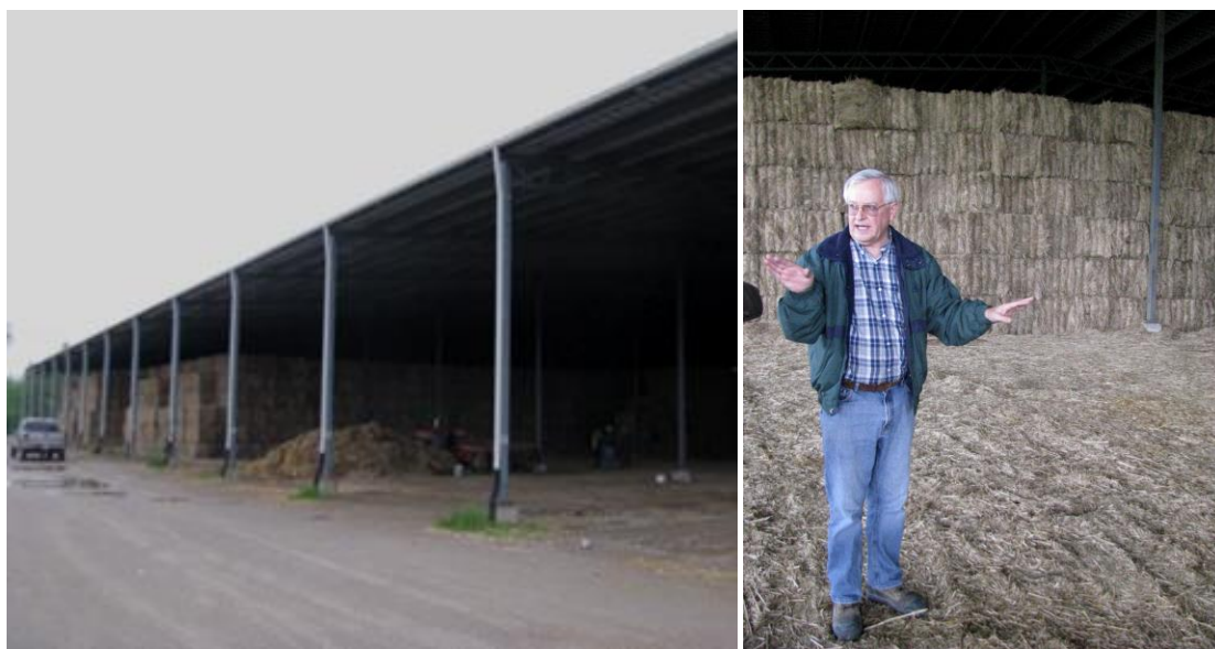
Figure 41. and Figure 42. Don Nott of Clinton Ontario explains his switchgrass metal storage shed facility. Bales are stacked 6 high and switchgrass straw is spread on the floor on top of the crushed gravel.
