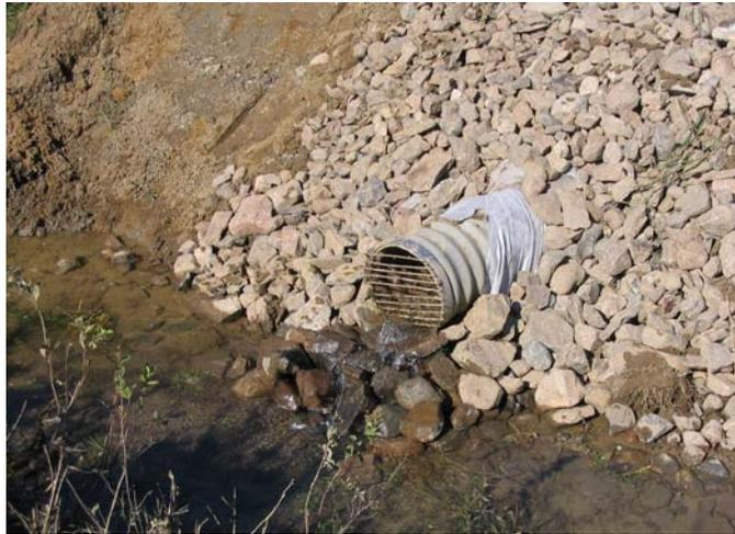
Photo 1: Drainage outlet with removable grate
