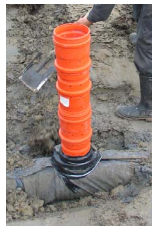
Connecting the inlet well to the drain
