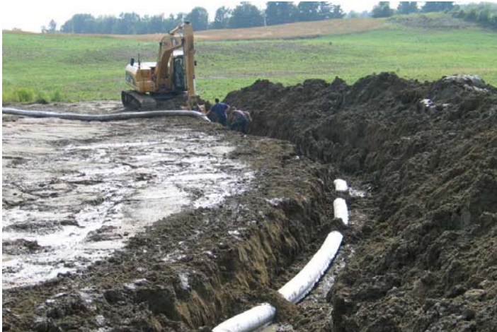
Excavating and installing the drain.
