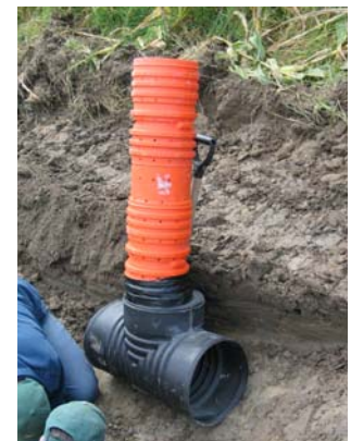
Installing an inlet well on a T-connection
