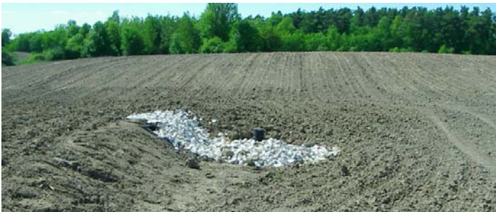
Inlet well with berm
