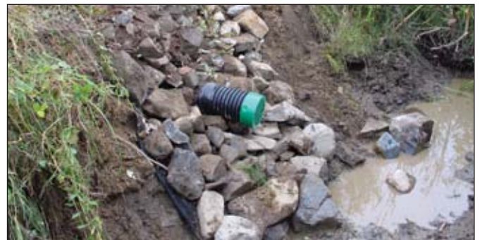
Photo 13: Erosion protection at a drain outlet Source: Mikael Guillou, MAPAQ
