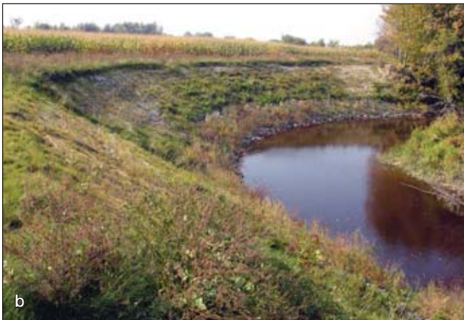
Photos 5 (a, b): Installations in a bend Source: Mikael Guillou MAPAQ
