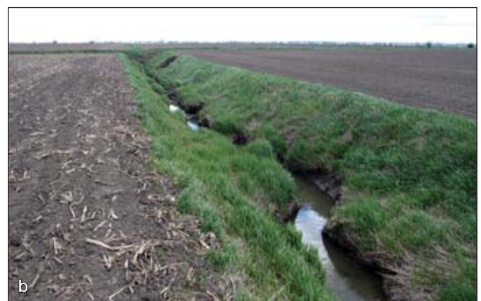
Photos 6 (a and b): Downcutting Source: Luc Lemieux and Mikael Guillou, MAPAQ
