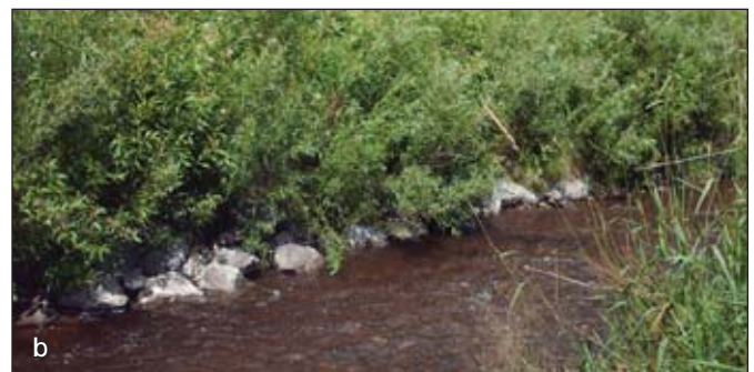
Photos 16 (a and b): Bank stabilization Source: Victor Savoie, Ghislain Poisson, MAPAQ
