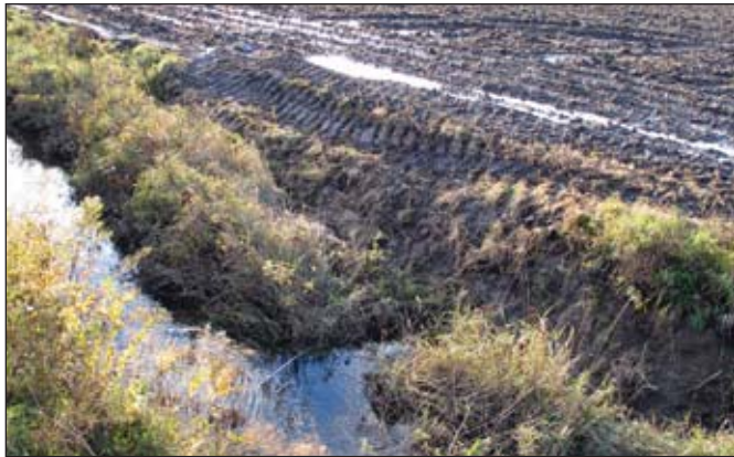
Photo 17: Failure caused by an excessive load Source: Mikael Guillou, MAPAQ
