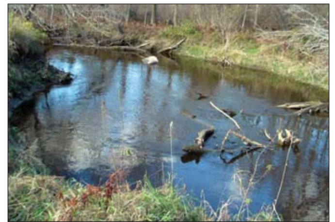
Photo 10: Bank erosion caused by an obstruction in the streambed. Source: Victor Savoie, MAPAQ
