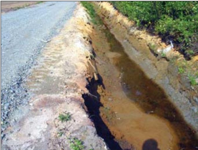
Photo 3: Piping caused by excavation of a stream in soil with an elevated water table Source: Victor Savoie, MAPAQ
